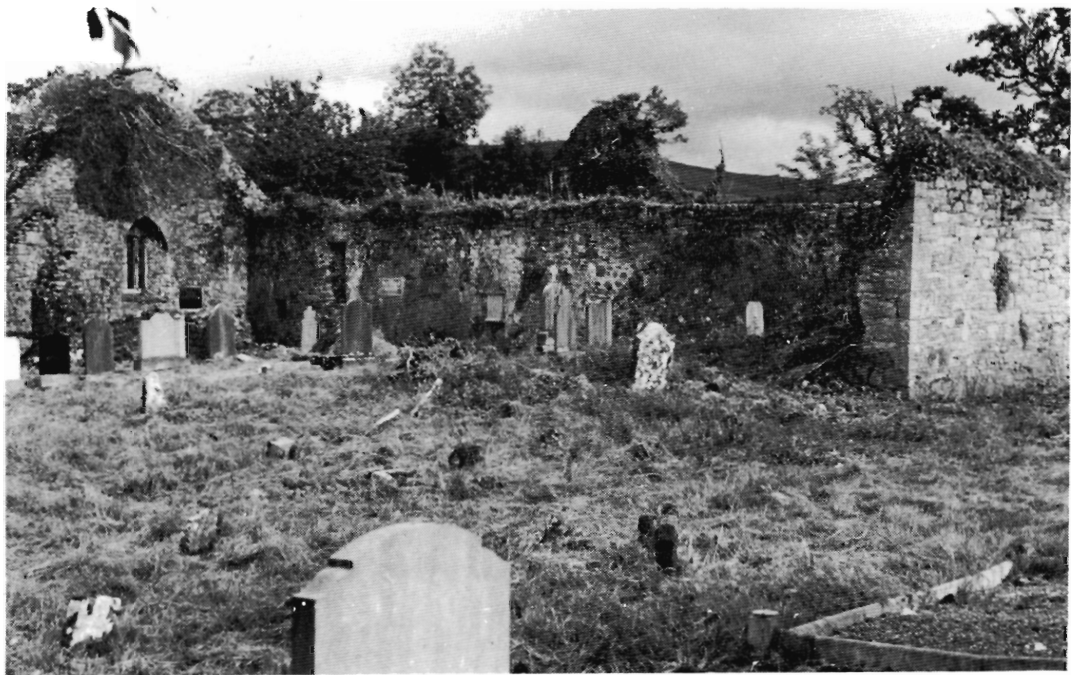
Fig. 3 Dolla Church from North-West before cleaning and reconstruction.
